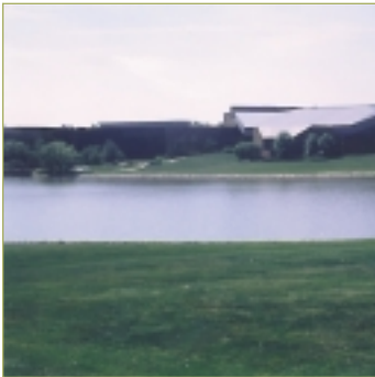
Fig.#32 The church and the storm-water pond immediately in front.
