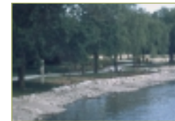
Fig.#65 The rip rap and the obvious ability of geese to tread right through. This rip rap is neither high nor dense enough to prevent geese from moving from the water to the grass.
